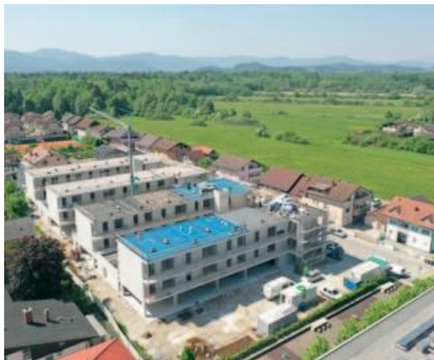
Figure 10: Dolgi most, Ljubljana, neighbourhood, aerial view, May 2022 (Matevž Lavrinc, s.p.)
